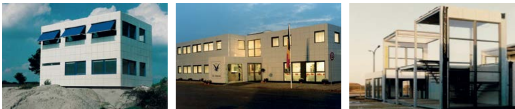
Figure 4.3. Left picture, the final design of the MAX60 in 1988 in Markelo and the middle picture in Breendonk, Belgium. Right picture shows also a frame turned placed as stairway
