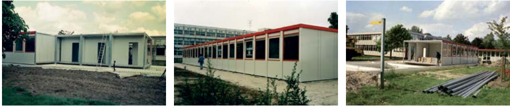
Figure 4.2. Assembly of the prototype of the MAX60 semi-permanent modular construction system on the campus of Eindhoven University of Technology in 1987. This building is still in use even in 2016!
